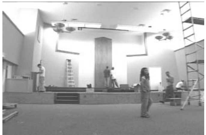
Church members help dismantle the fifth-floor chapel.
