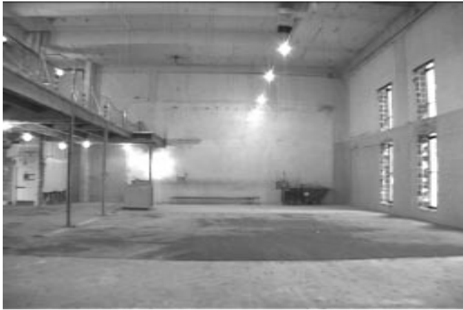
Fifth-floor construction where the terrestrial and celestial rooms of the Temple were built. The space housed racquetball courts when the building was first built in the 1970s.
