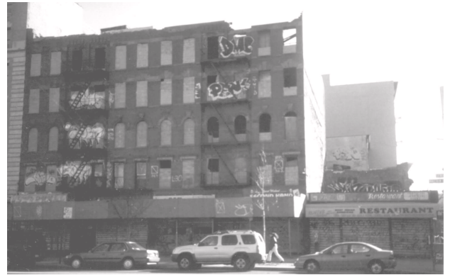
The site purchased for the new Harlem building
